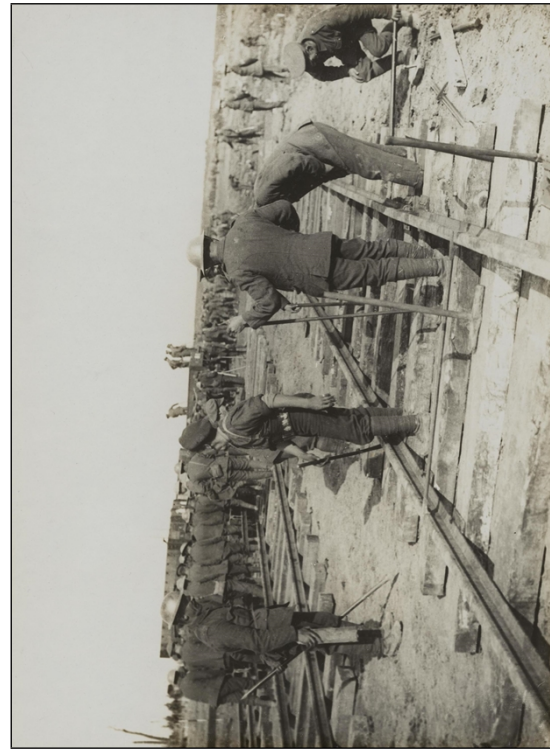
Fig. 8.1.10. Troops of the Royal Engineers laying track at the southern corner of Bernafay Wood. This is probably the west end of Trones Wood station. September 1916. Notable in a number of photographs is the use of "picaroons" (a Canadian tool similar to a boathook) to position the sleepers. Photo: AWM H08925
